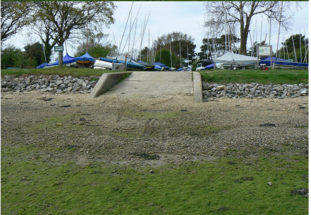
Cobnor Slipway (NP)
